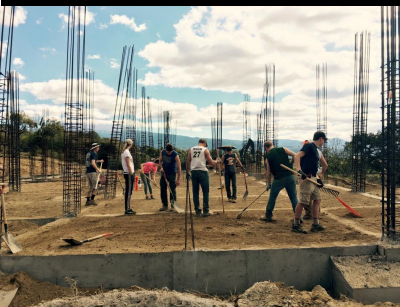
Smoothing the floor
