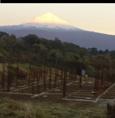
The filled foundation...ready for cement!
